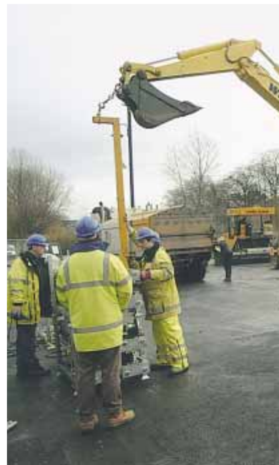
River Severn, Frankwell, Shrewsbury, September 2002
