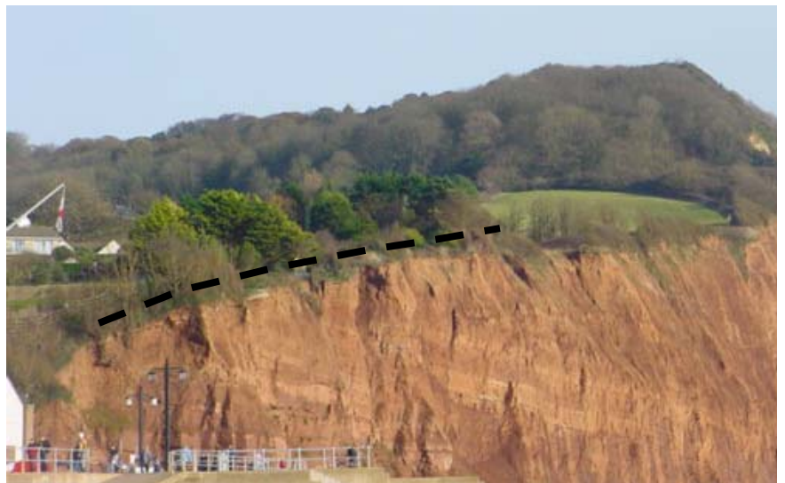
Figure 2 Line of the missing footpath on Salcombe Hill
